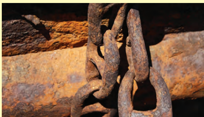
Fig 11.6. Rusting of iron
