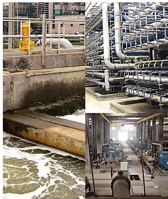
Fig. 8.12. The desalination plant at Minjur, Thiruvallur D.t.,
