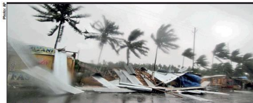
Cyclone Fani flattened roadside shops in Puri on Friday morning
