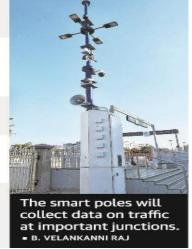
✓ The smart poles will have a rain gauge, public address system, camera and equipment to monitor pollution.
